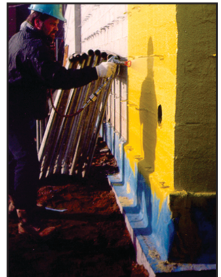
Above: Rub-R-Wall Airtight applied with pressure spray.
