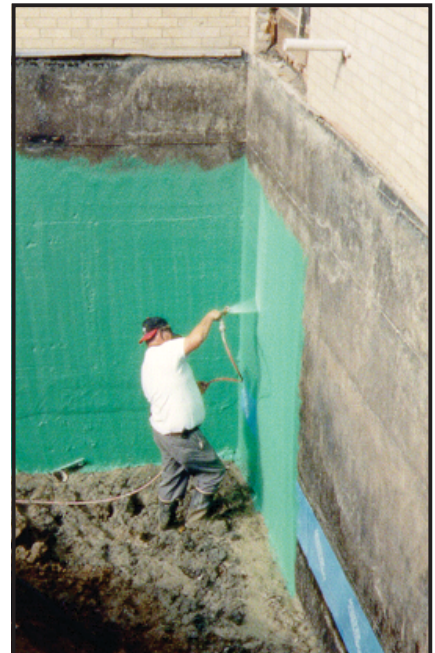
Above: Rub-R-Wall installed in retrofit application.
