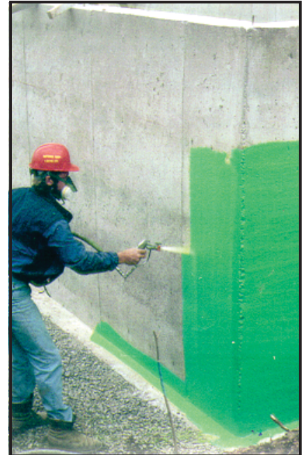
Above: Rub-R-Wall applied with pressure spray.
