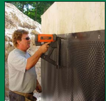
Wrap-N-Drain installation on a poured concrete foundation.
